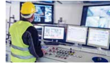
Activated by Control Room
