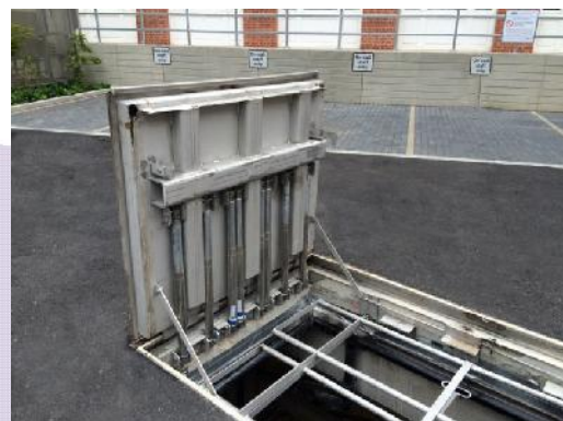
Grade 304 Stainless Steel Kent Multi-Paver installed in St. Barts Hospital, London (England)
