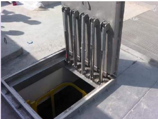
Grade 316 Stainless Steel Kent Hinged Multi-paver installed in Lusail City (Qatar)
