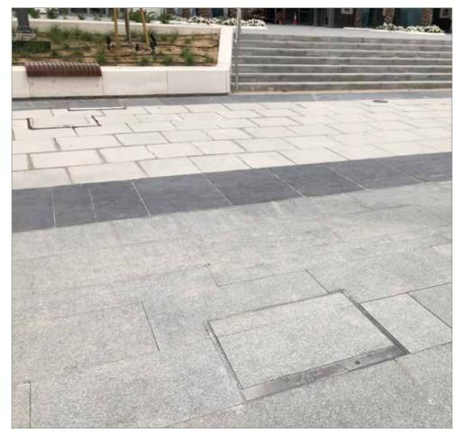
This box is used where there are multiple carts with heavy power requirements. Widen the box to add a strip of Data. Deepen the Box to use > 1nr 63 Amp 3 Phase Power.
